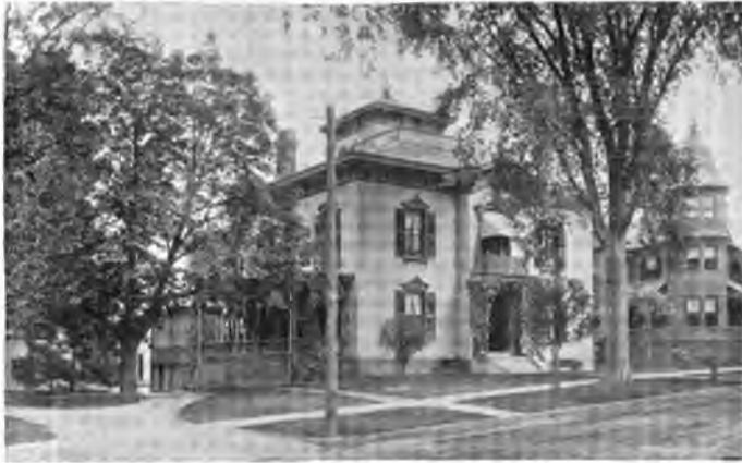
RESIDENCE OF MAYOR VAN PATTEN.
